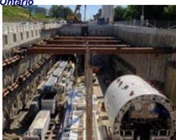
The ECLRT project is broken up into two contracts. The first contract, currently being constructed by the joint venture of Obayashi / Kenaida / Kenny, has completed their first two tunnel drives between Keele St. and Allen Rd., utilizing two CAT EPB TBMs. The two TBMs were removed, repositioned, commissioned and have resumed mining once again on the balance of the tunnels between Allen Rd. and Laird Dr.
