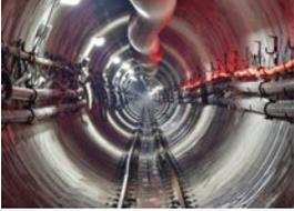
Tunnelling on Metro Vancouver's Port Mann Water Supply Tunnel Project was completed in July 2015. The project consisted of two slurry wall shafts, each approximately 60 m deep and located on either side of the Fraser River, connected with a 1 km long, 3.5 m diameter tunnel. Excavation of the tunnel was carried out using a CAT EPB TBM; construction was undertaken by the McNally-Aecon Joint Venture.
