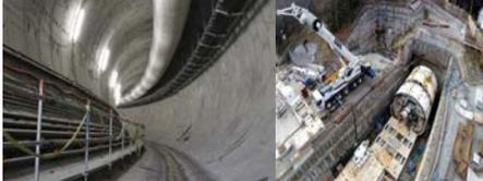
The Evergreen Line Rapid Transit Project is an 11 km extension to Greater Vancouver's rapid transit system. The project includes a 2 km long, 10 m diameter bored tunnel. The design-build-finance contract was awarded to EGRT Construction and the tunneling work is being conducted by SNC-SLI Joint Venture. The tunnel was excavated with a CAT EPB TBM – boring was completed in November 2015.
