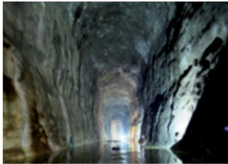
Jurong rock caverns (JRC) are located on Jurong Island and is Southeast Asia's first commercial underground facility for the storage of liquid hydrocarbons such as crude oil and condensate. "JRC" located 150 meters below the ground is able to optimize land use by saving up to 60ha of aboveground land, ensuring safety and security of the products in
