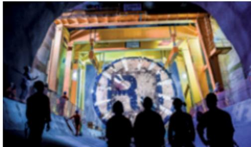
The shield-driven tunnel of metro line 4 in Rio de Janeiro (Brazil) has an approximate length of 5.2 km. the excavation was performed using a hybrid earth pressure balance shield with an excavation diameter of 11.51 m and passed through complex geology that
