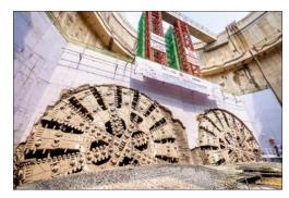
innovative solutions to cope with harsh ground conditions and hydrostatic pressure of 5bars at tunnel face (55m below sea level). The first 630m of excavation were also operated by a 17.63m diameter TBM (world's largest TBM), which was then reconfigured as a 14m diameter machine. 41 sub-sea cross passages were also constructed by mini TBM. The first breakthrough was completed on 27 February 2019 and the overall cost of works is estimated at €2.36bn.
