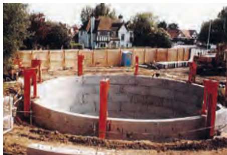
Figure 2 : Caisson sinking using jacks (Auld, 1997)
