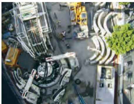
Figure 14 : Vertical shaft sinking machine VSM9000 constructing an urban shaft in Naples, Italy (Herrenknecht, 2020).
