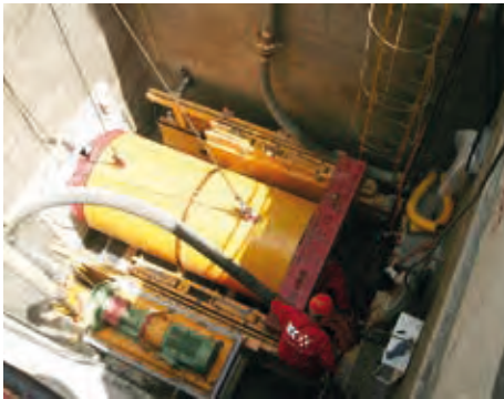
Figure 15 : Micro tunnel work shaft of Tehran's Western Sewage Canal (Mohammadi, 2020).
