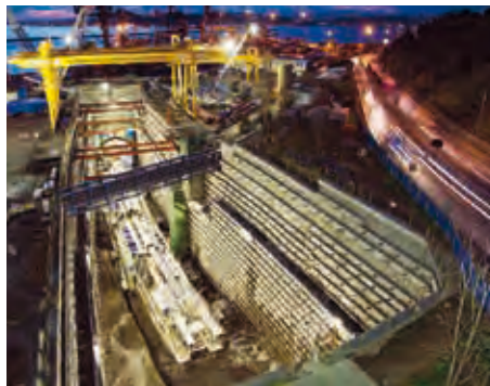
Figure 17 : Launch shaft for a Mixshield TBM at the Eurasia Tunnel on the Asian side of the Bosphorus, Istanbul (Herrenknecht, 2020).
