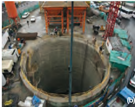
Figure 12 : (a) rectangular service shaft of Tehran's Metro Line 7 at Sanaat Square (Mohammadi, 2020) and (b) circular access shaft of Tehran's Metro line 6 at Vallsar Square (Mohammadi, 2020)
