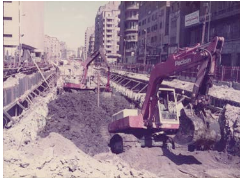
Open Excavation in Main Streets Close to Buildings & Traffic for
