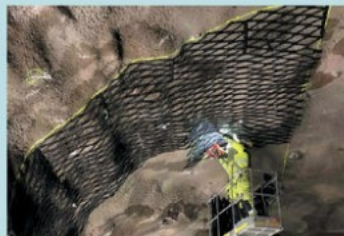
Above: Installation of innovation drainage mesh as an alternative to an internal driphed - alternative to standard Norwegian approach PHOTO CREDIT: ALUN THOMAS
