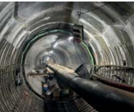
Below: Tunnel steel lining and welding in a hydropower tunnel. Underground projects are integral components of hydro projects and water storage reservoirs
