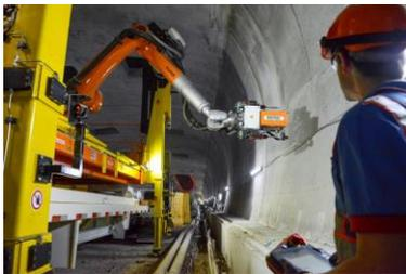
Advance in construction technology has enabled longer and larger tunnels to be built, and hence more E&M services are being installed along the tunnels to provide ventilation, lighting, security, communication, and fire service etc. There is an increasing demand, for construction workers, to install the E&M services and cladding, in particular, drilling anchors and installing permanent utility containment system including cable brackets and cable trays.
