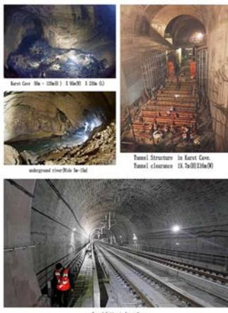
The project takes place in a section of Yujingshan Mountain Tunnel that encounters a giant 1.08 million m<sup>3</sup> karst cave hall and 18km long underground river (on the Chengdu-Guiyang High-speed Railway Line). The major part of the project was the construction of a tunnel crossing a giant karst cave and underground river.
