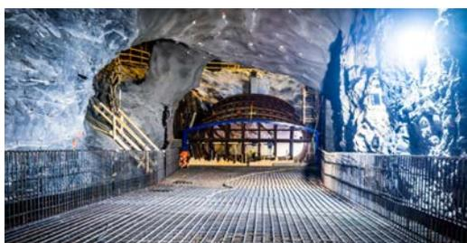
Nedre Otta Hydropower Project (Lower Otta HPP) is situated on the Otta river, one of the tributaries to Lågen river that further connects to Glomma, which is the longest river in Norway. The scope of works is the construction of an intake structure with a 200 m<sup>2</sup> trash rack area and two intake gates, 10.1 km unlined headrace and tailrace tunnel (90 m<sup>2</sup>), surge tunnels upstream and downstream, Powerhouse 65,000 m<sup>3</sup> with 15,000 m<sup>3</sup>
