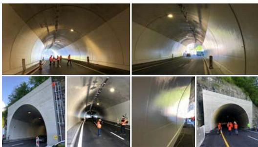
This project consists in the removal of part of primary lining, installation of drainage & sealing systems, final lining with self-compacting concrete, construction of verges incl. drainage, renewal of road surface, installation of electrical equipment.
