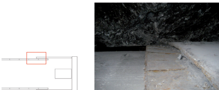
Figure 22 : Shield jamming due to squeezing rock [36]
