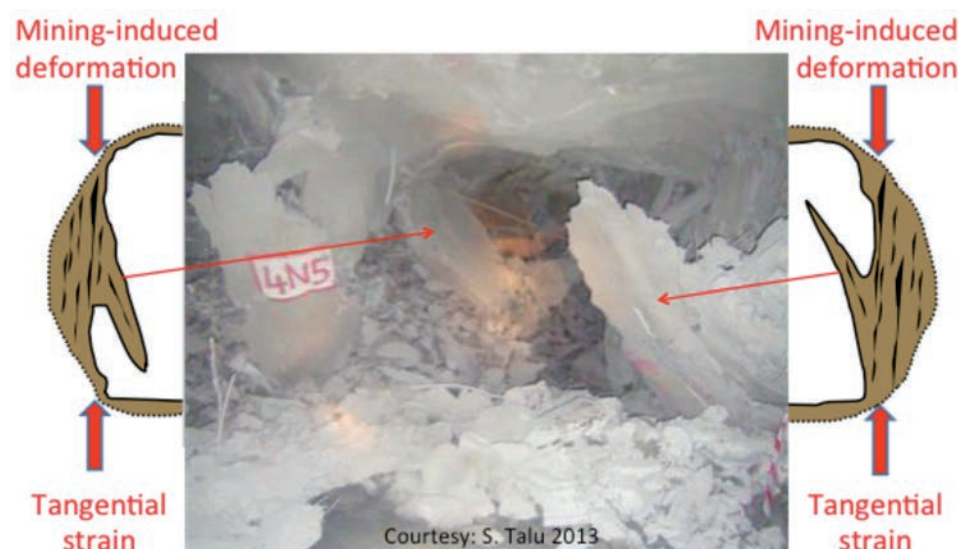
Figure 24 : Failed bull nose supported with bolts, mesh and shotcrete (Photo courtesy S. Talu).
