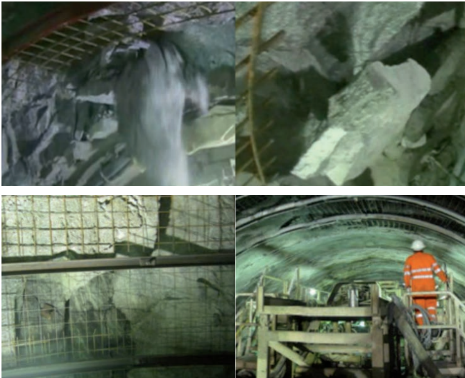
Figure 1 (top) : Rock “raining” from finger shield behind TBM and (bottom) steel arches “flying” without contact with tunnel roof (Photos courtesy: TAT consortium 2004)
