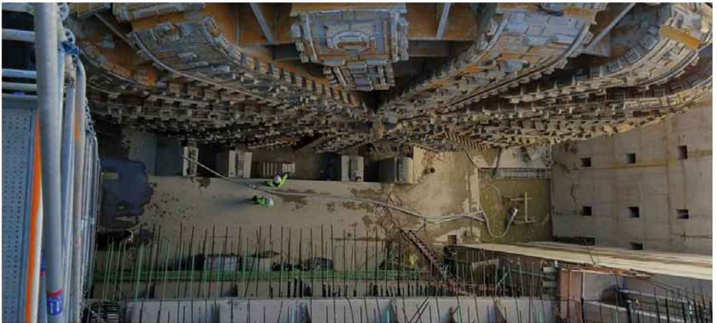
Figure 40 : Alaskan Way Viaduct Replacement EPBM in exit shaft.
