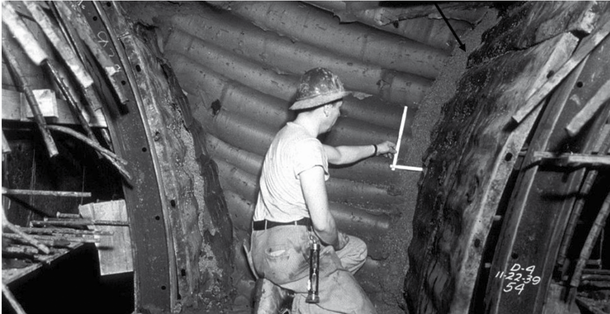
Figure 3 : Filling gaps with pea gravel between the excavated clay surface and the liner plate: Large gaps and delays in filling were a major source of ground loss.
