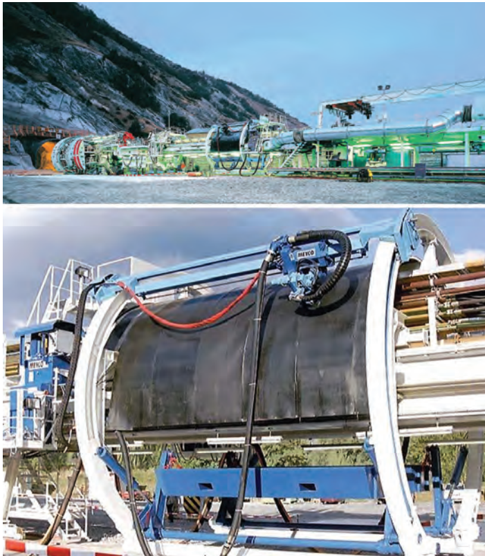
Figure 6: MEYCO Sprayed concrete robot running on ring beam behind TBM cutter head on the Lötschberg tunnel site, Gotthard Base Tunnel, Switzerland (Source: Meyco)
