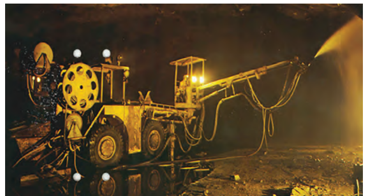
Figure 27: Furuholmen spraying robot on a CAT 944 carrier from seventies. (photo: T. Furuholmen)
