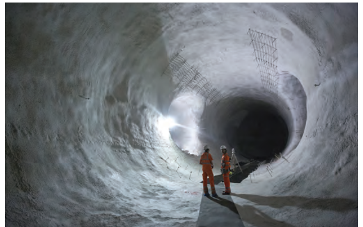
Figure 7: Circular geometry primary Sprayed concrete linings in excess of 40 cm thick for urban tunnels at 30m below surface (Source: Crossrail Ltd, London)
