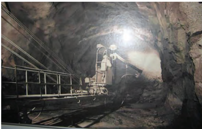
Figure 25: Stabilator dry spraying robot from 1960s (photo Ola Woldmo)
