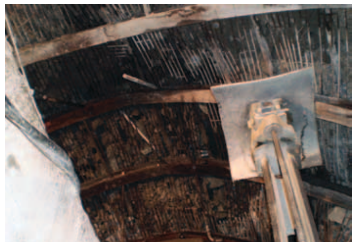
Figure 17. Steel McNally slats containing rock bursting in the tunnel crown
