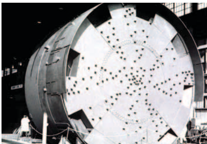
Figure 9. Compressed air TBM at the Paris RER Metro
