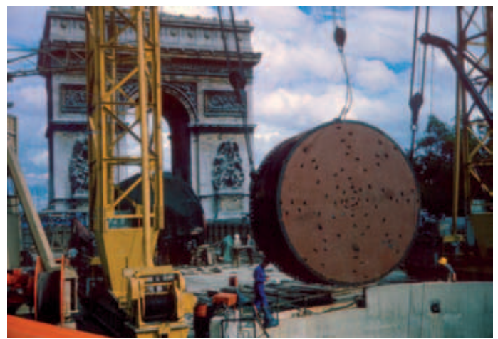
Figure 10. Lowering the cutterhead (Arc de Triomphe in background)
