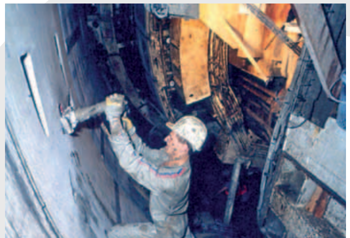
Figure 12. Setting Segments and Back-fill Grouting in the Channel Tunnel
