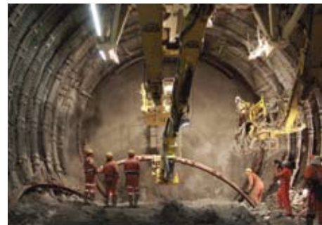
Steel arches (Gothard tunnel, © Alptransit Gothard)
