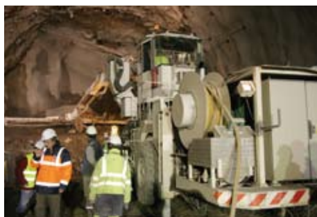
Drilling with a jumbo (Chavanne tunnel, ©RFF / www.imatec-photo.com)
