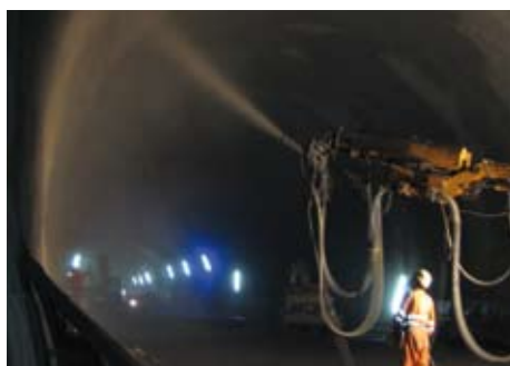
Robot sprayconcrete (Uetliberg tunnel)
