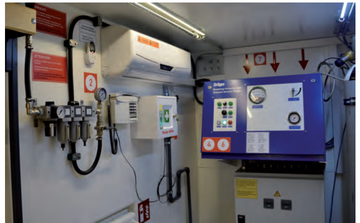
Filtration unit and air regeneration system – numerical symbols refer to steps in instruction manual
