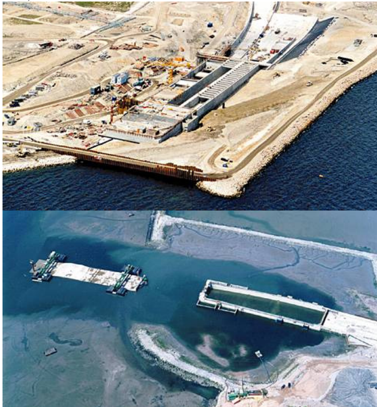
Approach structures can be built on the banks before, after or concurrently with the immersed tunnel, to suit local circumstances.
