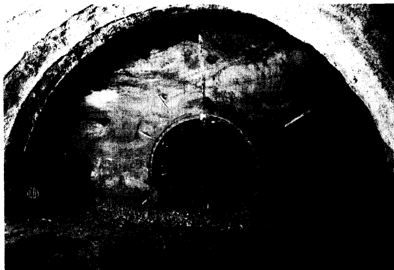
Figure 3. Preventive radial consolidation from TBM pilot bore in soft ground (Giemme 1989).
