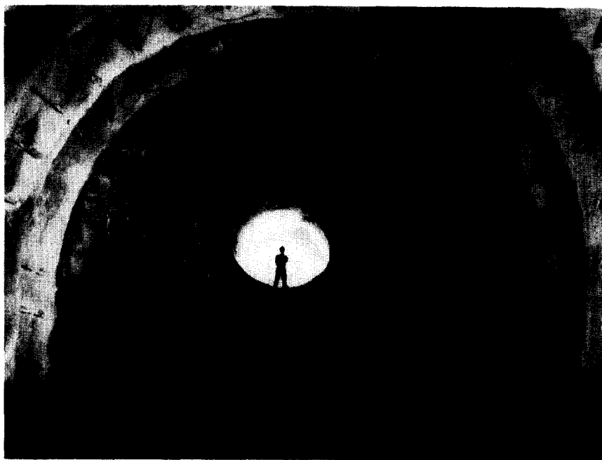
Figure 1. A TBM pilot bore (10m 2 ) in a railroad tunnel (95m 2 ) in a flysch rock mass (Leonardi 1987).
