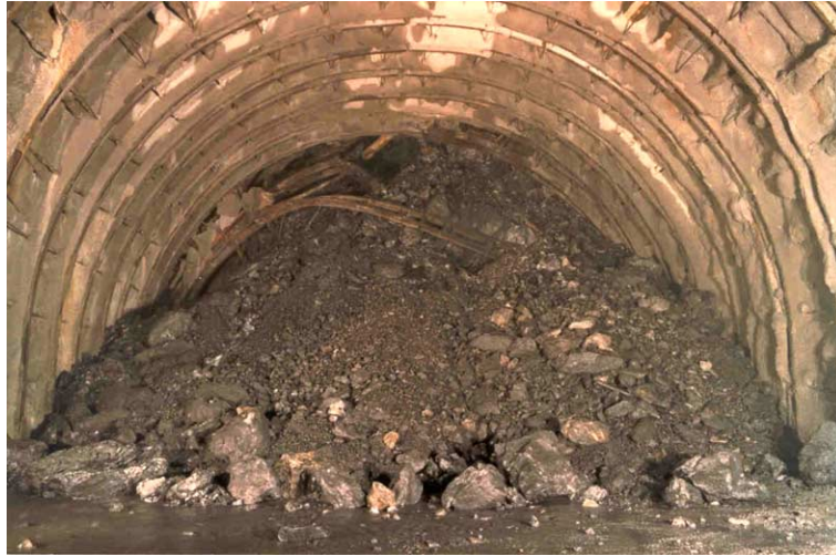
Fig. 6. Collapse due to a sinkhole in the crown of loosen material in a tunnel supported by steel arches and shotcrete.
