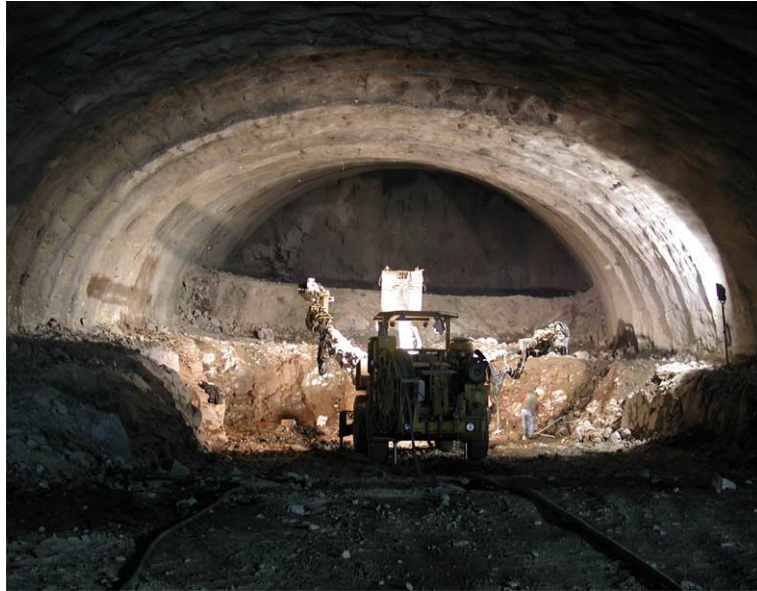
Fig. 4. Diversion in road tunnel, conventional tunnelling (Bolzano, Italy, courtesy S.Tua, Soc.It. Condotte d'Acqua).
