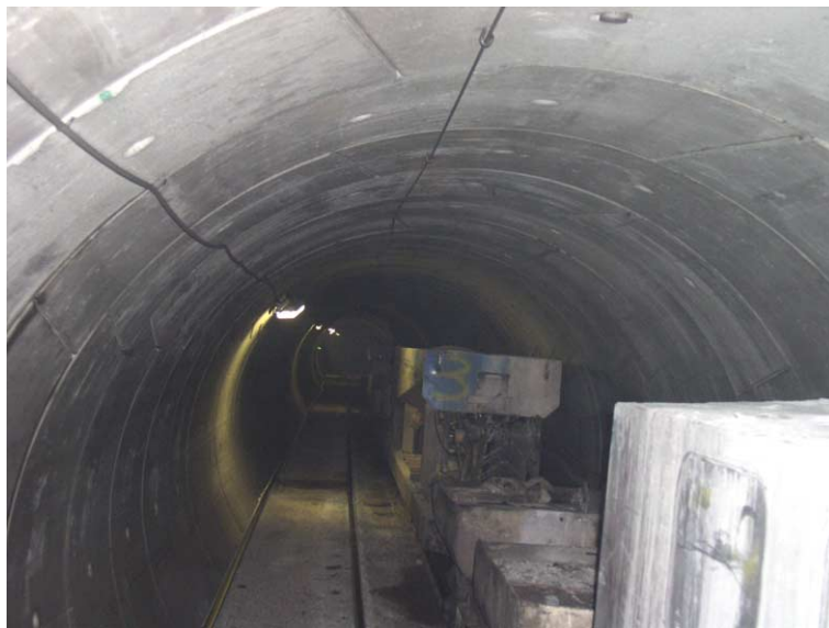
Fig. 5. Hydroelectric tunnel, mechanized tunnelling (Bormio, Italy, C. Oggeri with permission of M.Concilia, SELI).
