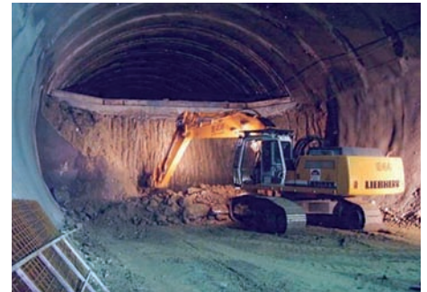
Mechanical excavation, top heading bench
