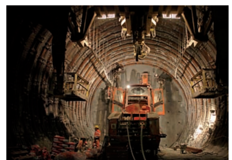
Conventional tunnelling in squeezing ground (full face)
