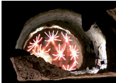
Drilling and blasting, full face
