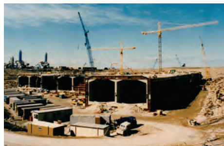
Figure 4 : Tunnel elements are constructed in the dry, for example in a casting basin, a fabrication yard or in a factory unit.
