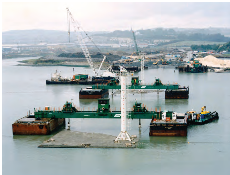
Figure 5 : Immersed tunnel element being prepared for immersion. Note the survey towers, one of which is used for interior access.
