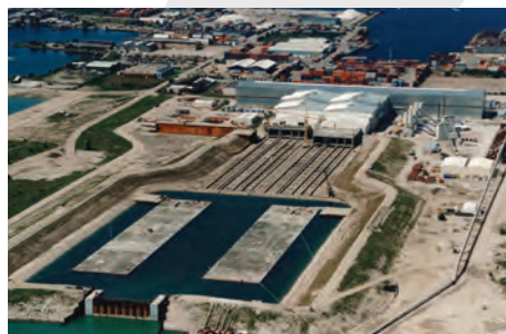
Figure 4 : Tunnel elements are constructed in the dry, for example in a casting basin, a fabrication yard or in a factory unit.
