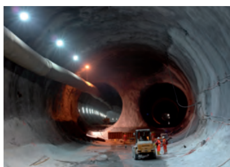
Figure 4 : - Top: Drilling jumbo working in a conventional tunnel drive. - Below: Tunnel bifurcation excavated by conventional tunnelling General description of the project development process © AlpTransit Gotthard Ltd.
