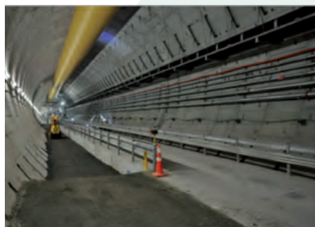
Figure 3 : Top right: Pipe-jacking tunnel as water sewer Lower right: Backfilling the gaps aside of an invert gallery in a large tunnel parallel to tunnel excavation © Babendererde Engineers
