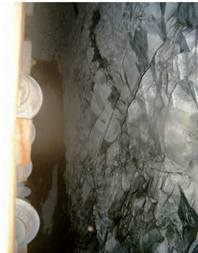
Tunnel face without any mark of disc cutter
