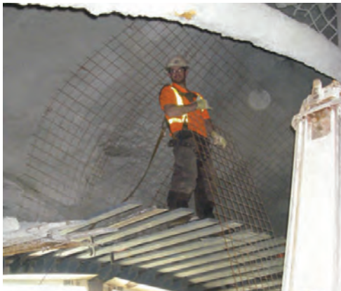
Over-break above the TBM
