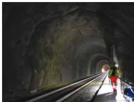
Figure 6 : Recently constructed PSCL tunnels in Norway. Right: The Holmestrand rail tunnel, constructed 2012-2015, portion in mixed face with soil and hard rock, with waterproof PSCL in the foreground and the interface to the traditional concrete segment waterproofing shield system. Left: Gevingås rail tunnel, constructed 2009-2011; meta-greywacke (meta clay/sandstone), groundwater table approximately 80 m above the tunnel crown, drained invert (Photos: Karl Gunnar Holter)
