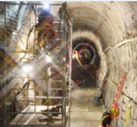
Installation of the rock support in a rock trap
