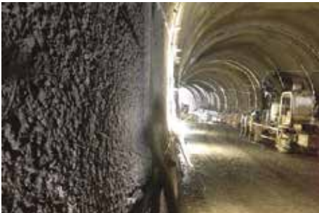
Applied macro synthetic fibre reinforced sprayed concrete in the driven tunnel.
