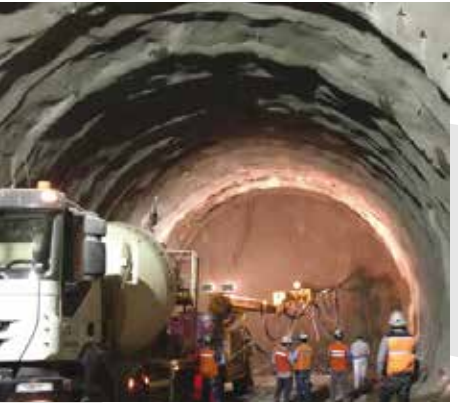
Spraying concrete at the tunnel face.
