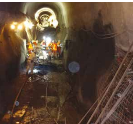
Excavation of a rock trap
