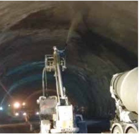
Serra do Cafezal T2, sprayed concrete lining.
