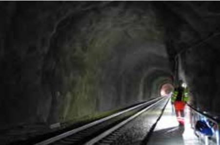
Central portion of the 4100 m long Gevingås railroad tunnel in central Norway, with permanent sprayed concrete and bonded spray-applied waterproofing membrane.
