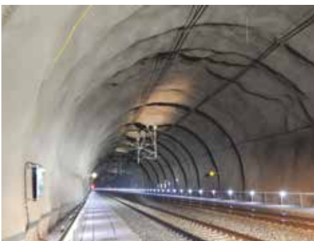
Figure 6 : Recently constructed PSCL tunnels in Norway. Right: The Holmestrand rail tunnel, constructed 2012-2015, portion in mixed face with soil and hard rock, with waterproof PSCL in the foreground and the interface to the traditional concrete segment waterproofing shield system. Left: Gevingås rail tunnel, constructed 2009-2011; meta-greywacke (meta clay/sandstone), groundwater table approximately 80 m above the tunnel crown, drained invert (Photos: Karl Gunnar Holter)
