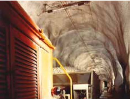
Vereina tunnel, single-track D&B section.
