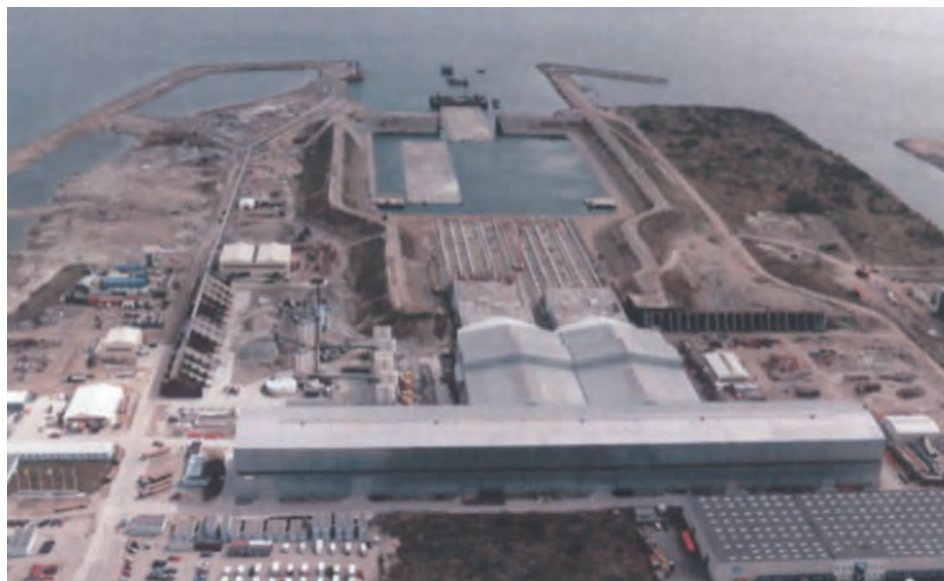
Figure 1 : Factory production site for Øresund Tunnel (Denmark)
