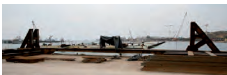
Figure 4 : Jacking frame - is hung beneath outboard end of element (Bosphorus Rail Tunnel).
