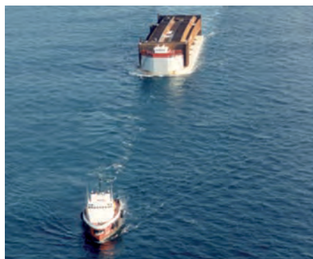
Figure 1 : Example of tunnel element being transported by semi-submersible barge.
