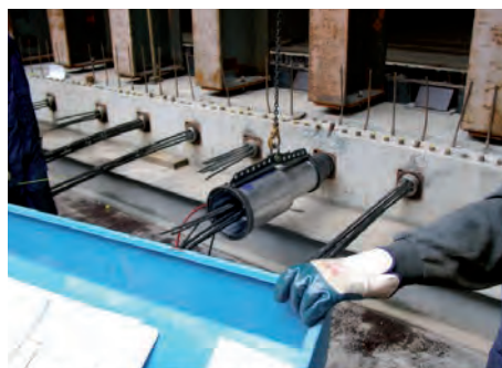
Figure 2 : Applying prestress with a hydraulic jack
