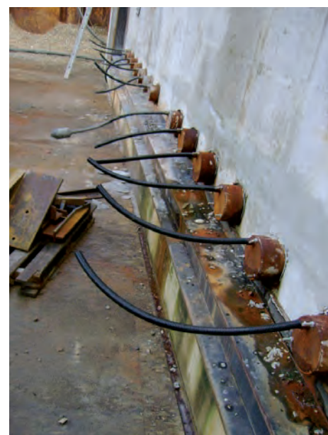
Figure 3 : Anchor heads after grouting
