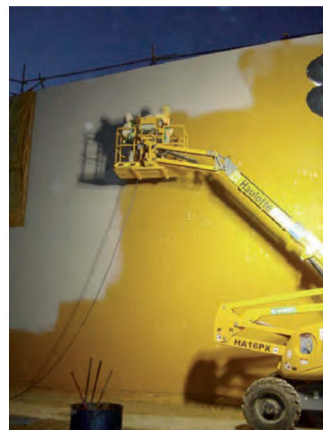
Figure 4 : Elastomeric polymer spray membrane
