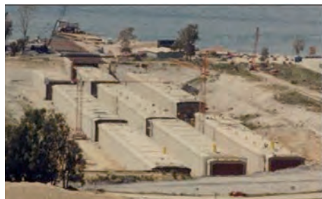
Figure 1 : The Aktio-Preveza tunnel has a spray applied membrane to the walls and roof, and a plastic membrane to underside of base
