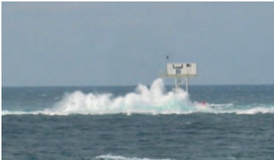
Figure 8: Wave loads on tunnel element during sea transport.
