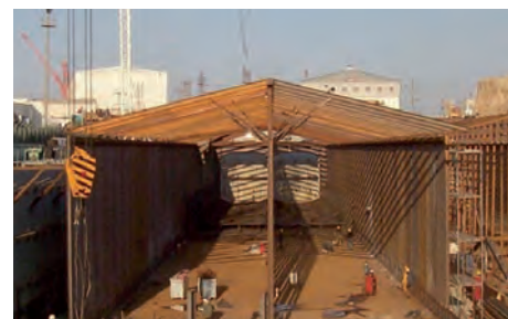
Figure 2 : Marmaray Tunnel steel membrane
