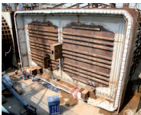
Figure 5 : Inboard end of element with central shear key and two guide beams (Bosphorus Rail Tunnel).
