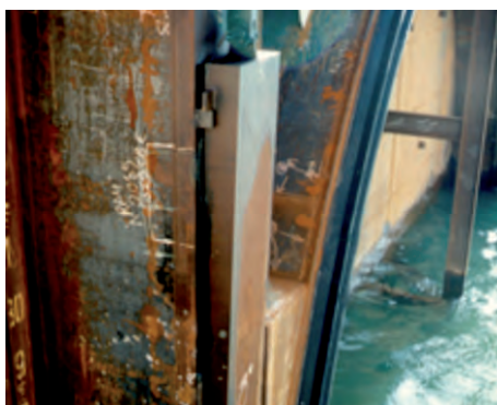
Figure 3 : Inboard joint showing movable wedge.
