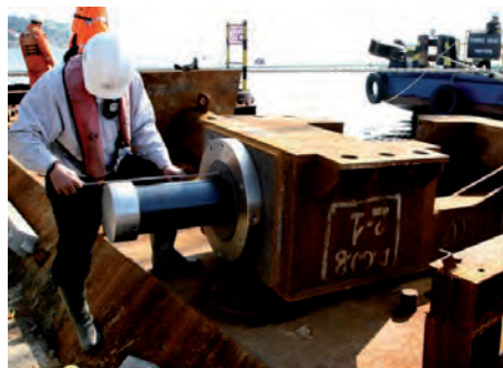
Figure 10 : An adjustment jack being installed.
