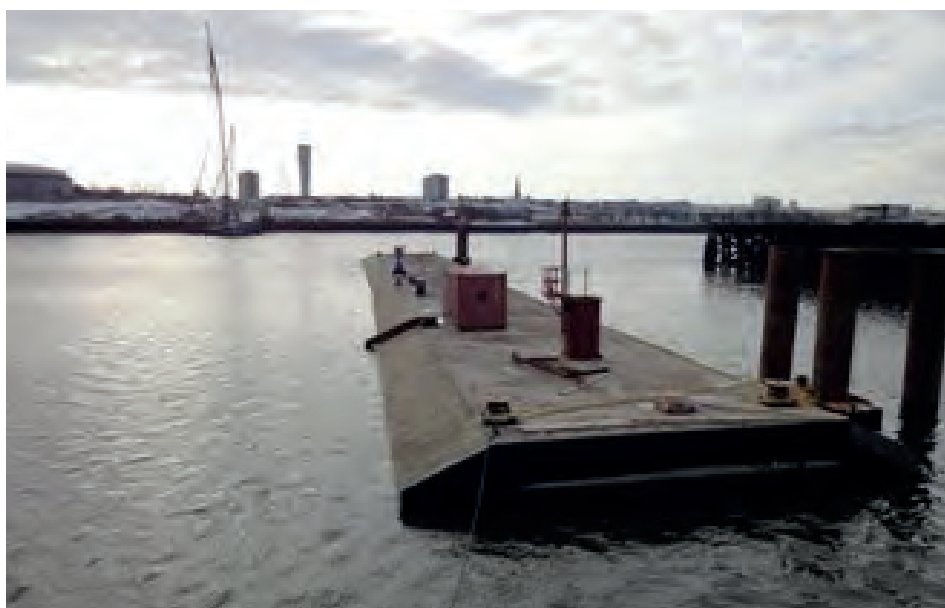
Figure 4: Tunnel element moored after transport at temporary parking location, near immersion location.
