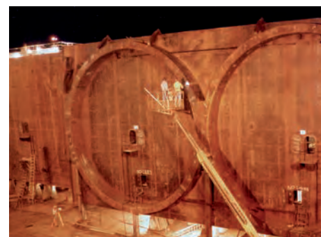
Figure 2 : Night survey validation of outboard face of a steel shell element.
