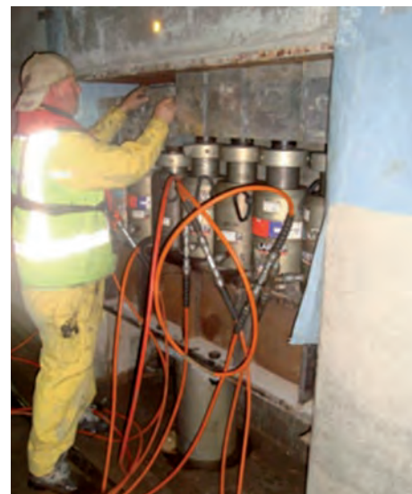
Figure 4 : typical secondary support assembly
