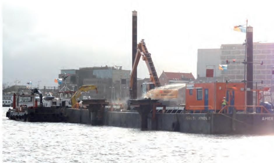
Figure 4 : Re-use of dredged material as trench backfilling material for the NZL Metro project in Amsterdam
