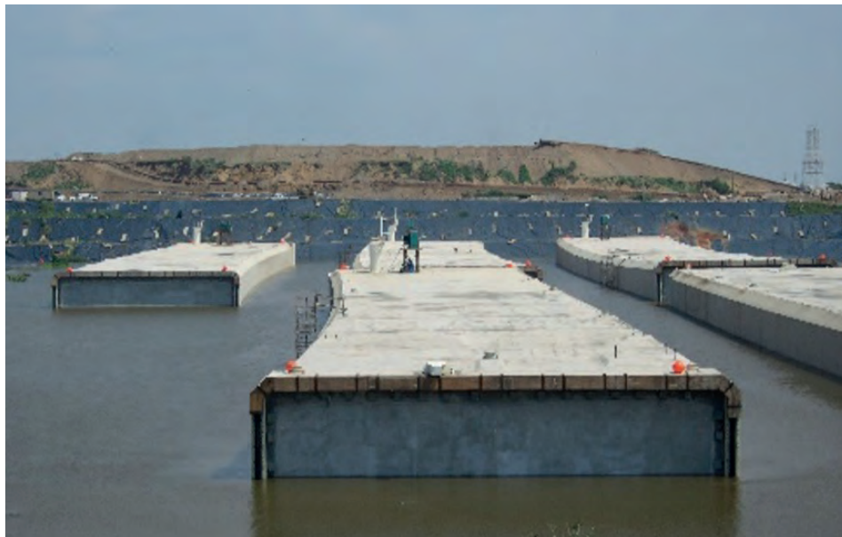
Figure 2: Elements are transported with tugboats.
