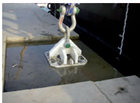
Figure 2 : Typical suspension lug
