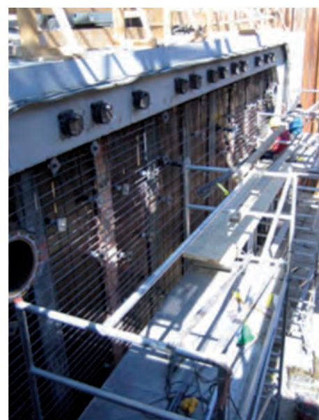
Figure 7 : Prestressing anchorages at end face of element
