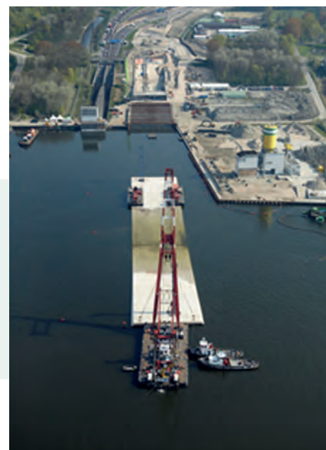
Figure 1 : Immersion operations next to existing immersed tunnel (left).
