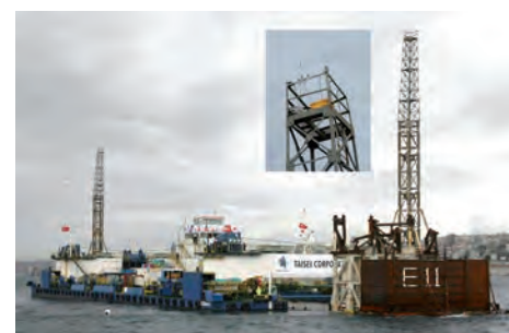
Figure 7 : GPS towers with inset showing arrangement of equipment on towers. (Bosphorus tunnel)
