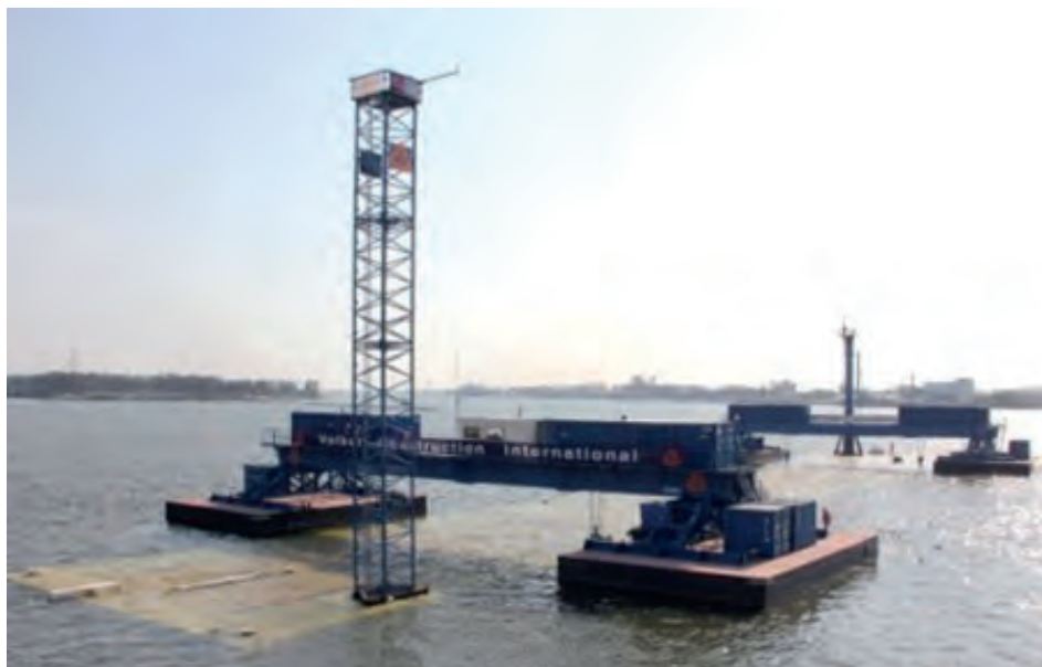
Figure 6: Lowering of a tunnel element through the waterline by catamaran.
