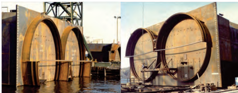
Figure 3 : Steel closure joint Fort McHenry Tunnel, Baltimore
