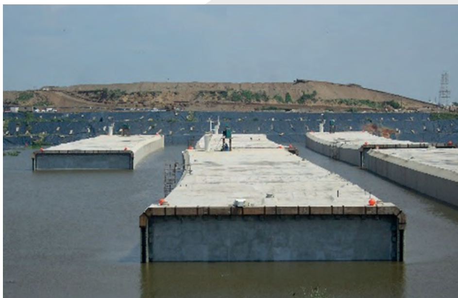
Figure 2: Inundation of the construction dock.
