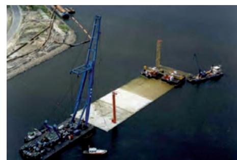
Figure 6 : Tunnel element with access shaft (red) and survey tower (yellow)
