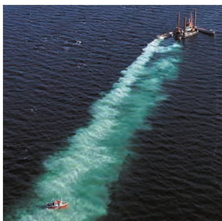
Figure 9 : Environmental monitoring of spill at Øresund Link project
