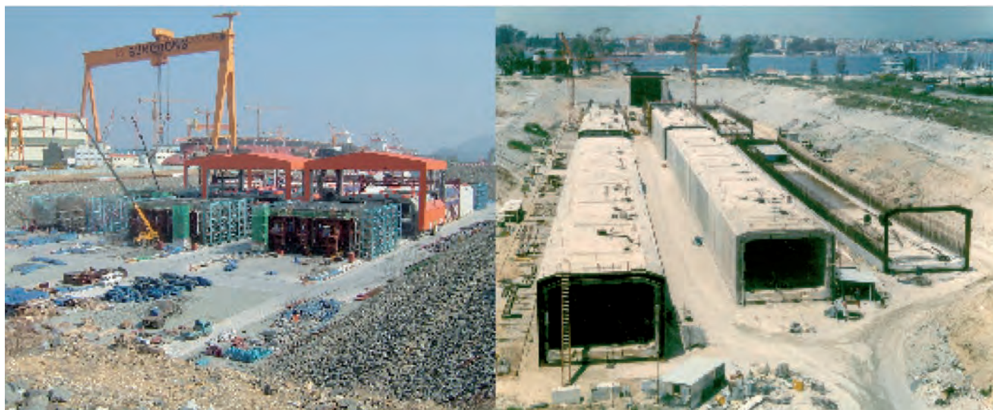
Figure 1 : Casting basins for Busan-Goeje, South Korea & Preveza-Aktio Greece
