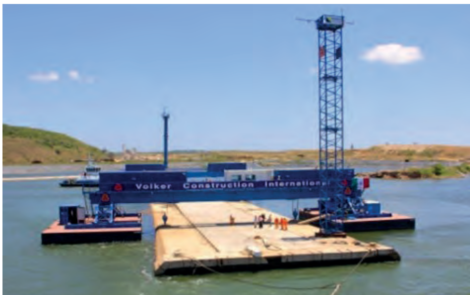
Figure 9: Horizontal positioning of an element before immersion.
