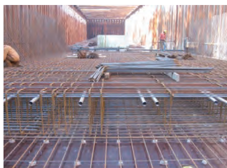
Figure 1 : PT ducts fixed into reinforcement cage
