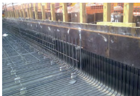
Figure 3 : T-lock plastic membrane
