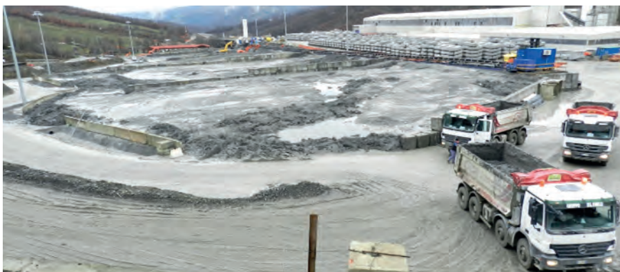
Figure 51: Sparvo Tunnel Project – Spoil Treatment (drying and mixing) Site and Off-Site Haulage
