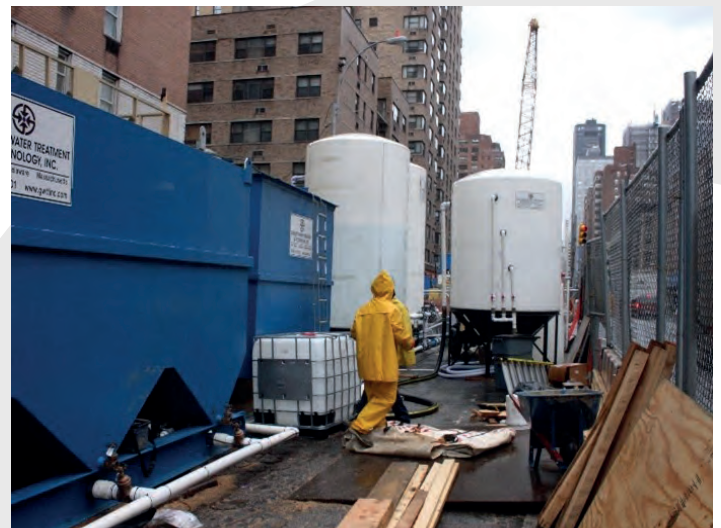
Figure 58: Second Avenue Subway – On-Site WTP
