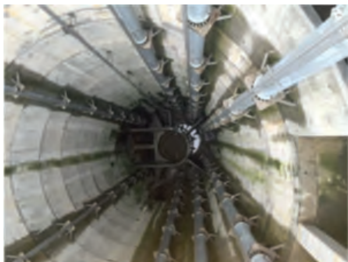
Figure 60: OARS Tunnel – Access and Pump Shaft Interior view of the access and pump shaft used for the TBM launch and tunnel spoil handling operations. (Courtesy of Kenny Construction)
