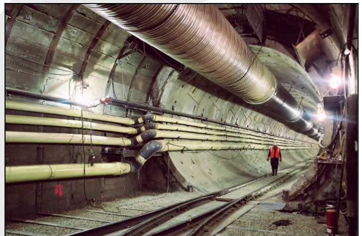
Figure 8: Arrowhead Tunnels Project – Cross-Section General arrangement of the tunnel cross-section showing utilities and spoil haulage (train) system.
