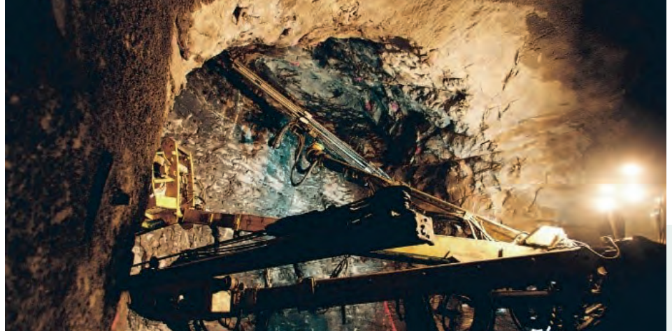
Figure 38: Second Avenue Subway – Adit Drill and blast operations at a full-face an Entrance adit connected to the Station Cavern.
