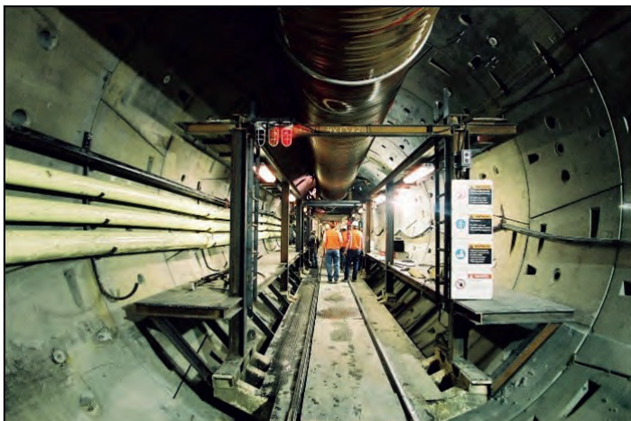
Figure 7: Arrowhead Tunnels Project – TBM General arrangement of the TBM trailing gear, utility systems, tunnel spoil haulage (train) system.
