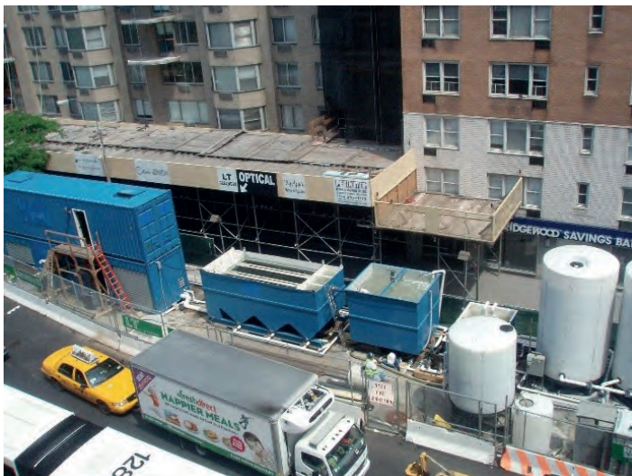
Figure 57: Second Avenue Subway – On-Site WTP
