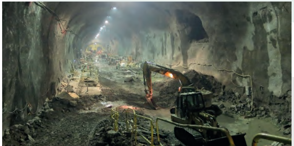
Figure 39: Second Avenue Subway – Station Cavern Lower-level drill and blast operations in the Station Cavern. Some invert concrete has commenced.
