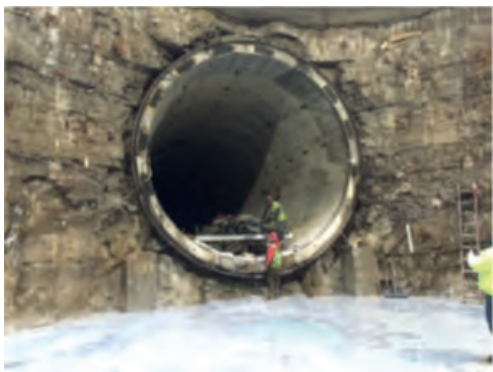
Figure 59: OARS Tunnel – Segmentally Lined View of the completed segmentally lined tunnels at Shaft 6 (upstream tunnel terminus). (Courtesy of Kenny Construction)
