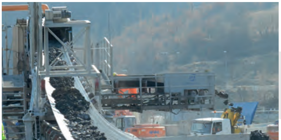
Figure 48: Sparvo Tunnel – EPB Tunnel Spoil Conveyor Tunnel spoil conveyor point of discharge at the surface storage and treatment area.
