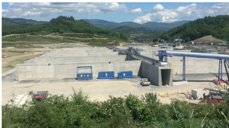
Figure 25: Santa Lucia Tunnel Spoil Storage Area Pre-construction appearance of the walled spoil storage area for the Santa Lucia Tunnel Project.
