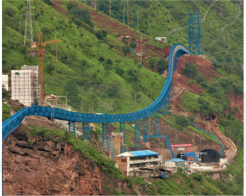
Figure 8 : Site installations and conveyors belt solutions at Jinping Hydropower Project, China (Marti Technik Ltd).
