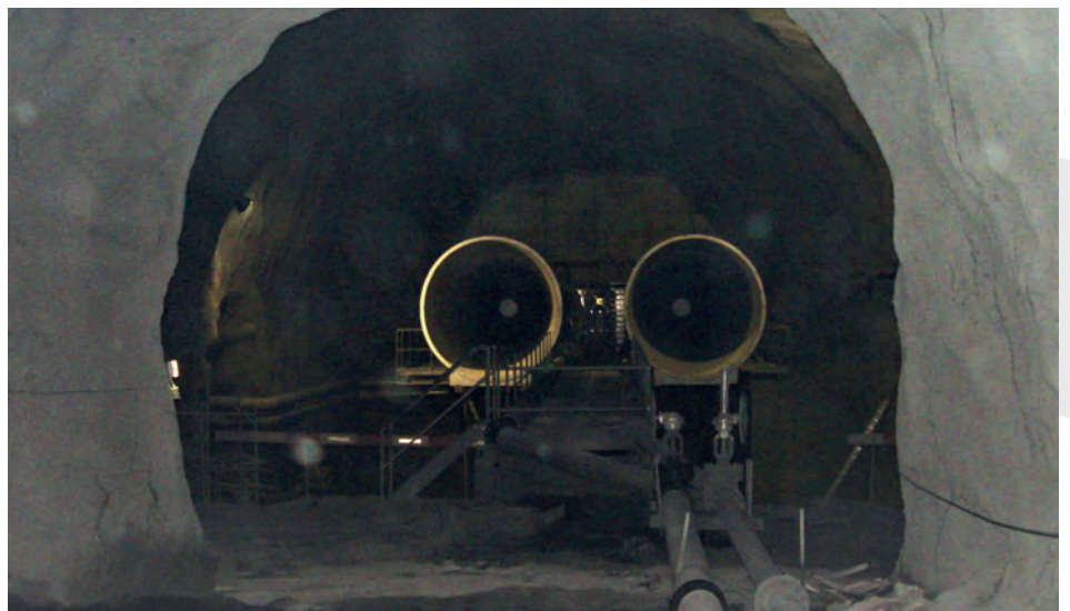
Figure 47 : Ventilation Installation (duct + dedicated gallery) at the bottom of Ferden (Lötschberg Base Tunnel) .
