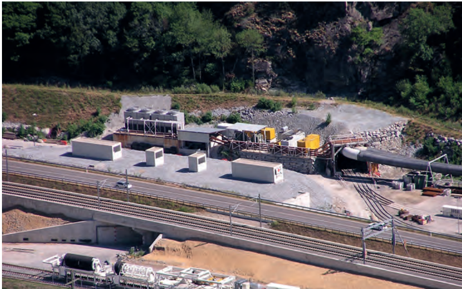
Figure 55 : Cooling installation at portal (Gotthard).
