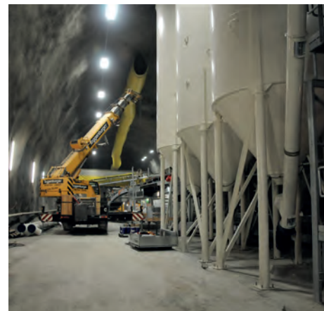
Figure 39 : Underground concrete plant, Ceneri Base Tunnel (Pini Group Ltd.).
