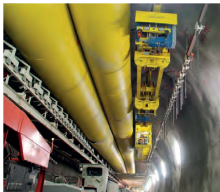
Figure 59 : Monorail and crown fixation with bolts and chains.
