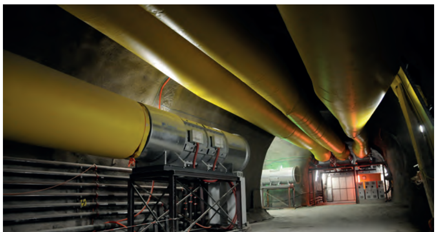
Figure 16 : Example of caverns for logistic installations (ventilation, de-duster, conveyor belt) in Faido.
