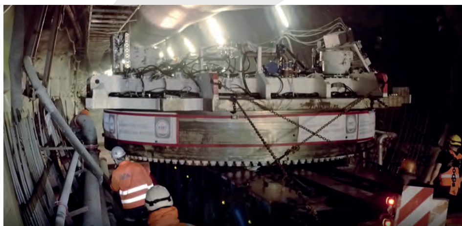
Figure 15 : TBM supply in restricted space, Brenner (courtesy BBT).
