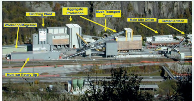
Figure 38 : Spoil handling facilities at Gotthard Base Tunnel south section (including spoil transport tunnel to final disposal).
