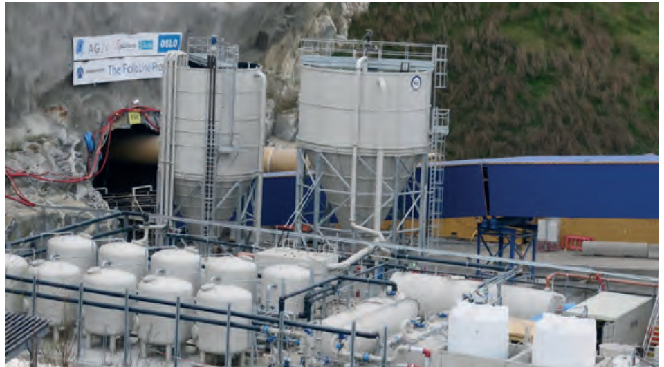
Figure 23 : Water treatment plant under construction, Follo line, Norway.
