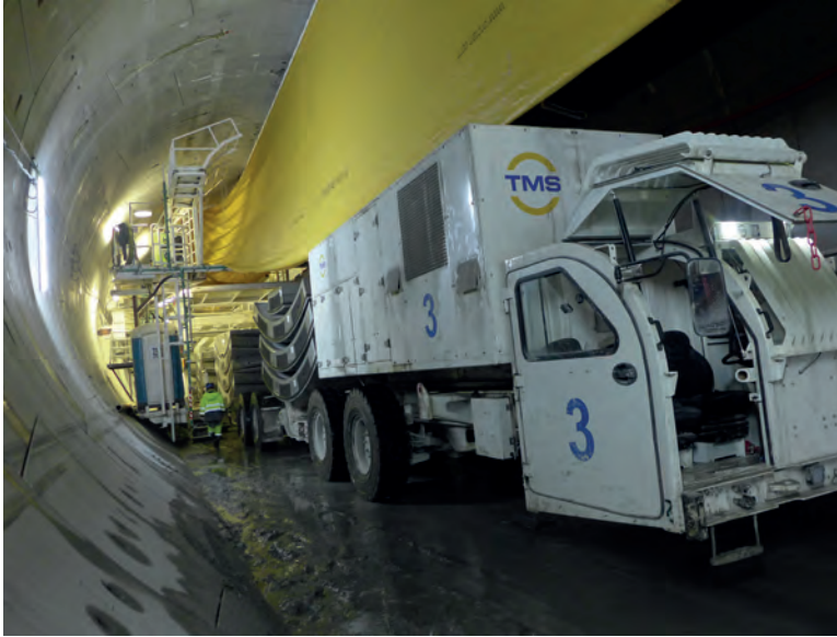
Figure 45 : Follo Line - Segments transported on MSV are de-loaded within the TBM (courtesy Bane NOR).
