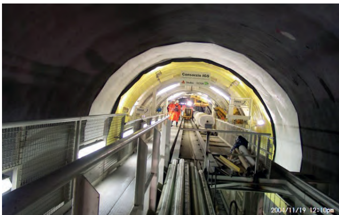
Figure 61 : Placing of waterproof membrane and reinforcement within the «WURM».
