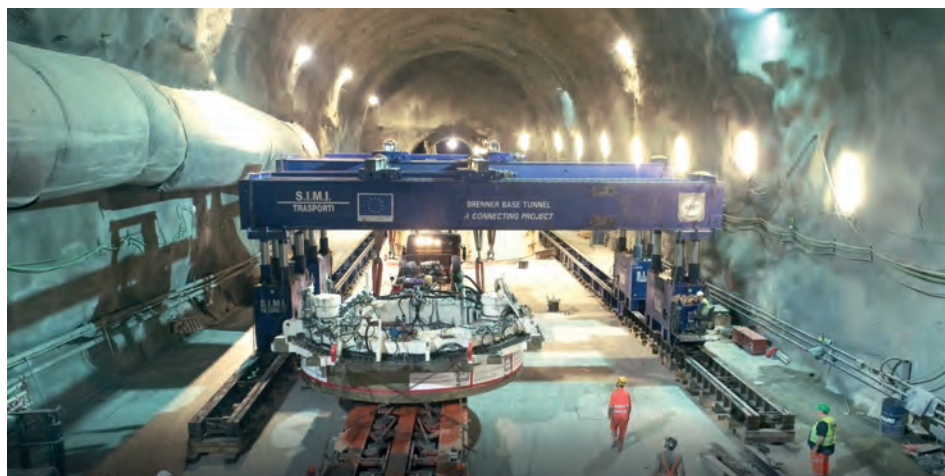
Figure 19 : Brenner Base Tunnel, TBM Assembly cavern (courtesy BBT)
