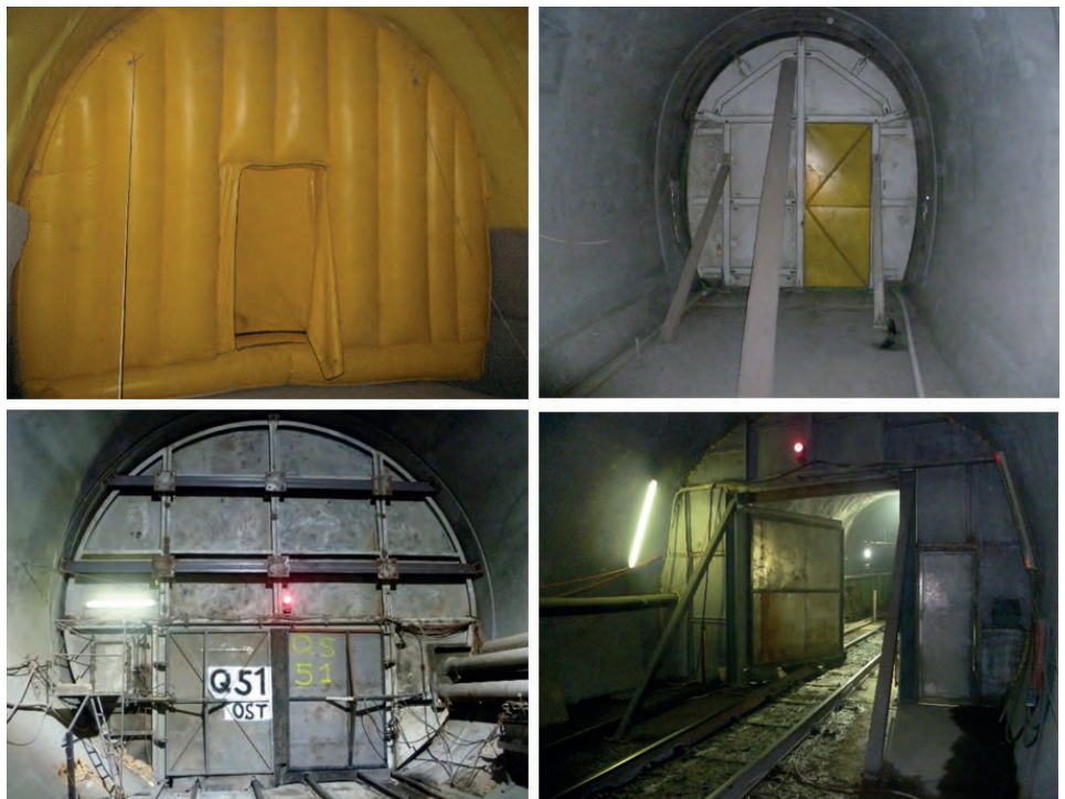
Figure 48 : Inflatable or fixed weather doors to close cross passages and main tunnel (Gotthard Base Tunnel).
