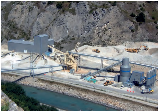
Figure 37 : Reuse of excavated material site, Modane 2005, (courtesy TELT).
