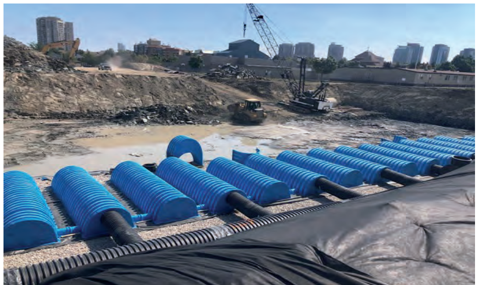
Figure 26: Stormwater chambers are installed under the City of Mississauga's Sandalwood Park. 5
