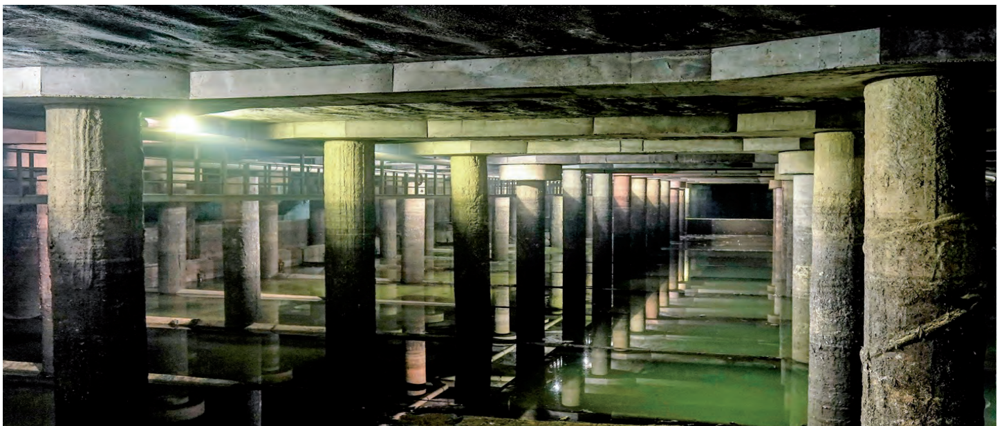
Figure 36: 400.000m 3 Storm water reservoir in Madrid, Spain.
