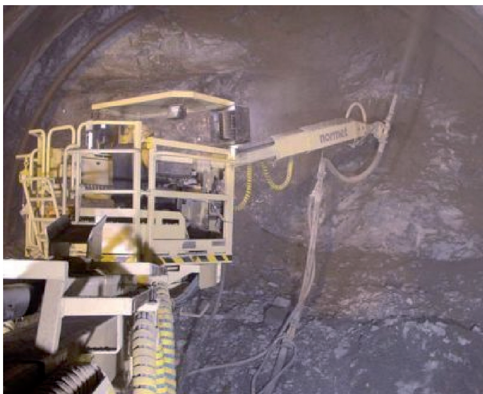
Photo 5: Concrete spraying, wet mix method.
