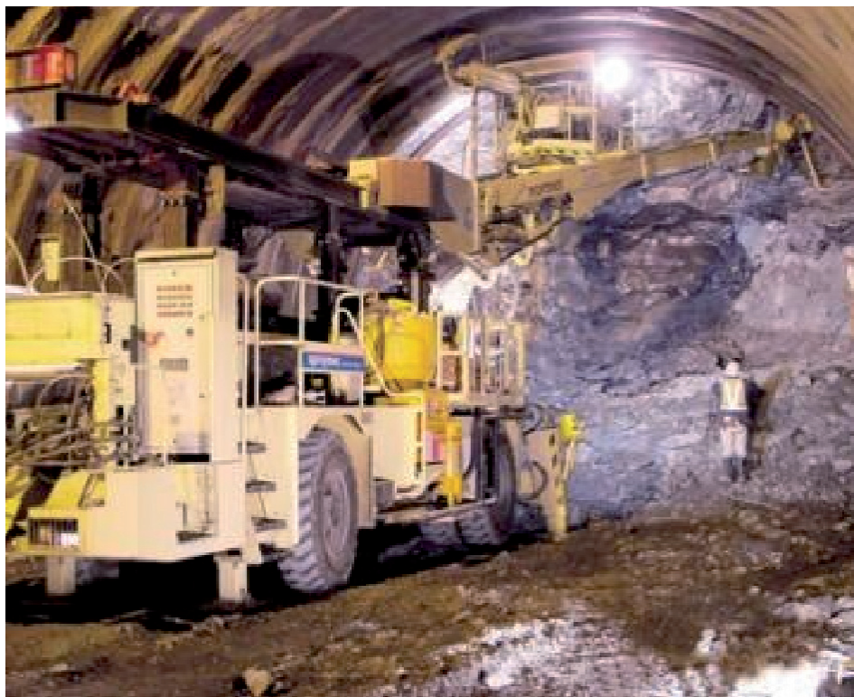
Photo 6: Concrete spraying, wet mix method, and arch installation.
