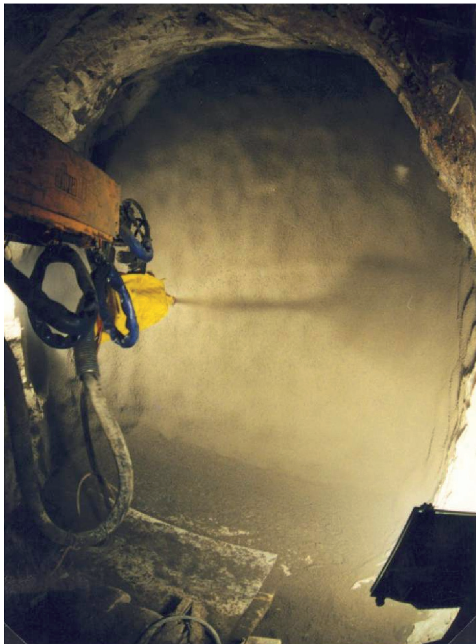
Photo 9: Application of steel fibre reinforces sprayed concrete in the gas reservoir Příbram – Haje in the Czech Republic (photo Vaclav Braun).
