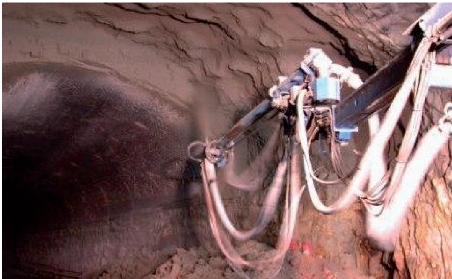
Photo 8: Steel fiber reinforced shotcrete being applied as primary support.
