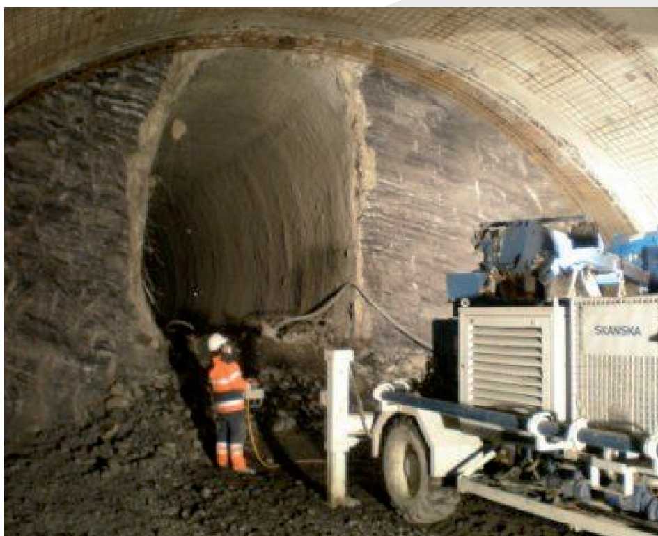
Photo 7: Application of the wet mix sprayed concrete in the Komorany road tunnel in the Czech Republic.
