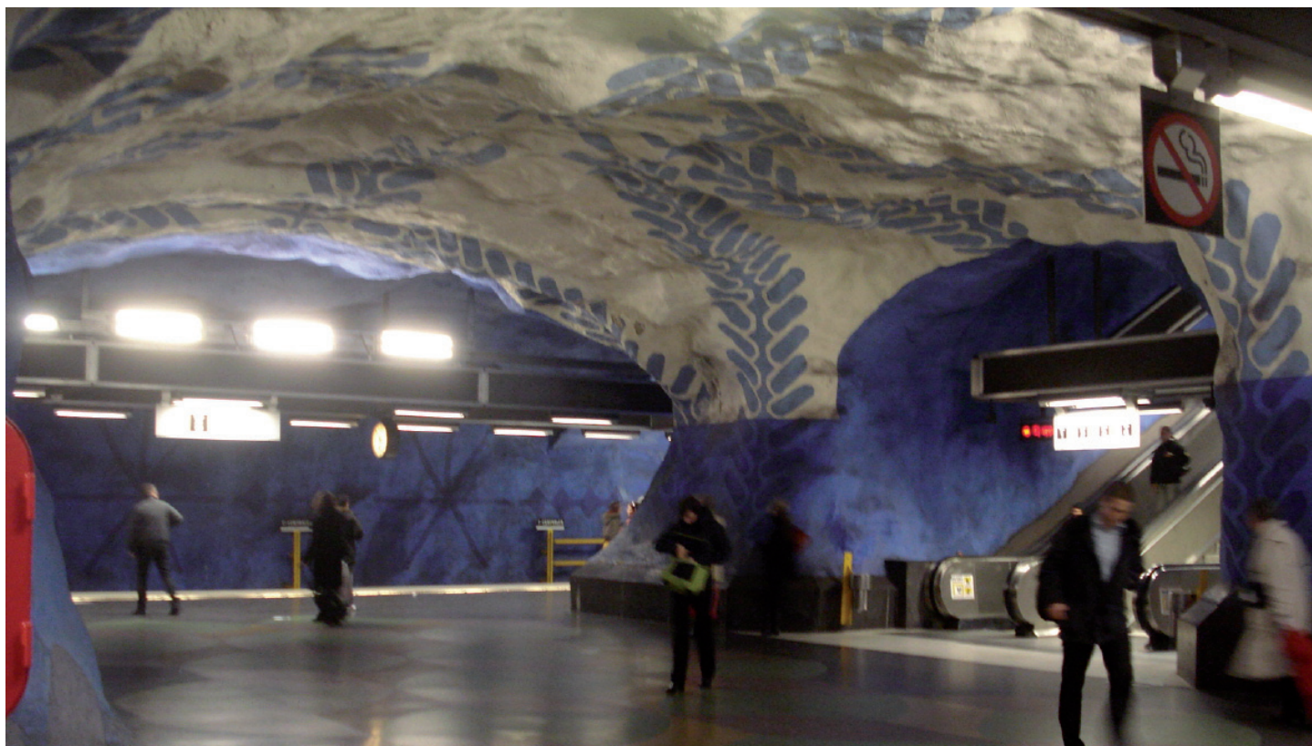
Photo 6: Final lining shotcrete for T-Centralen Station, Stockholm Metro.
