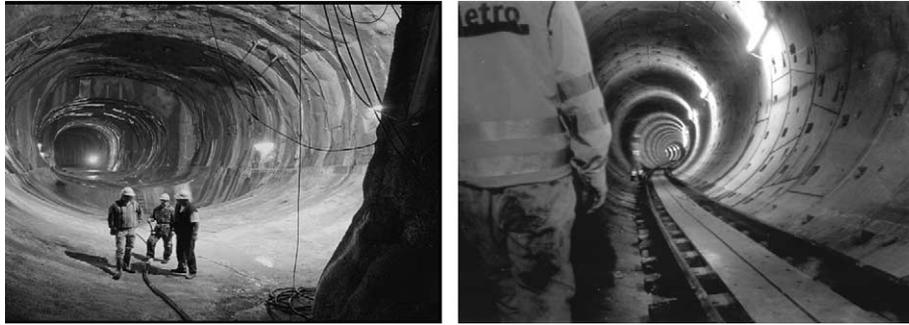
Fig. 8. Bifurcation cavern constructed by NATM (left) and running tunnel by TBM (right).
