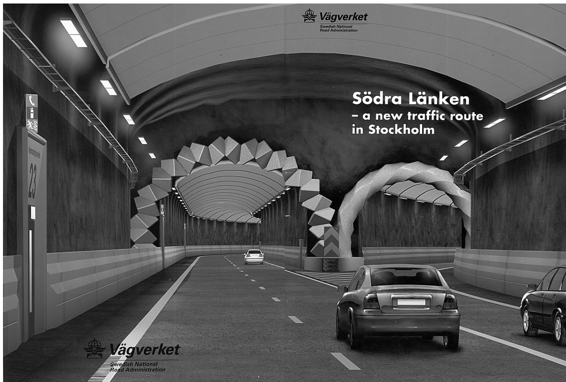
Interior of the Södra Länken road tunnel in Stockholm, Sweden (showing the light ceiling, the lightning, roch texture rock walls, amber distance markers, collision protection, emergency exits and the light-coloured asphalt) Total length of tunnel system including access tunnels 16.6 Km. Open for traffic October 24, 2004
