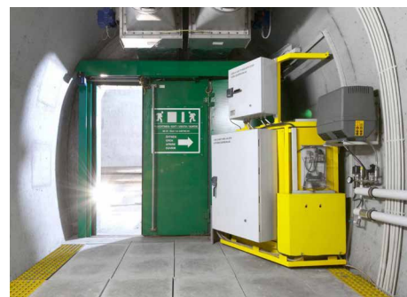
Figure 20: Double-leaf segment sliding door [19]
