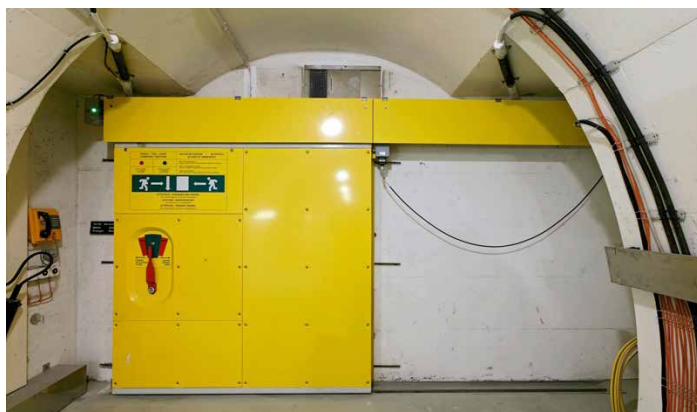
Figure 11: Single segment sliding door of Loetschberg Base Tunnel (view from inside the CP)
