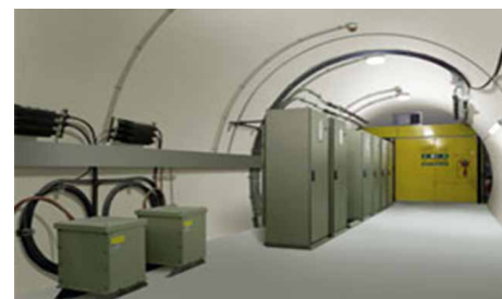
Figure 24: Cross-passage in Loetschberg Base Tunnel from rail tunnel (left) and inside (right)
