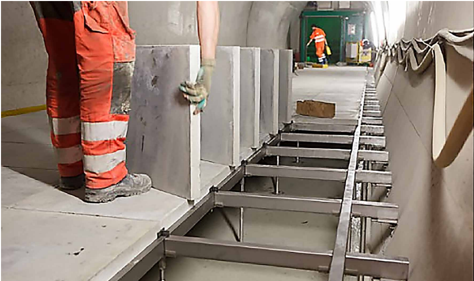
Figure 7: GBT false floor [source: ABAG Doppelboden]
