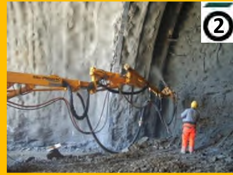
Sub Activity Group Sprayed Concrete
