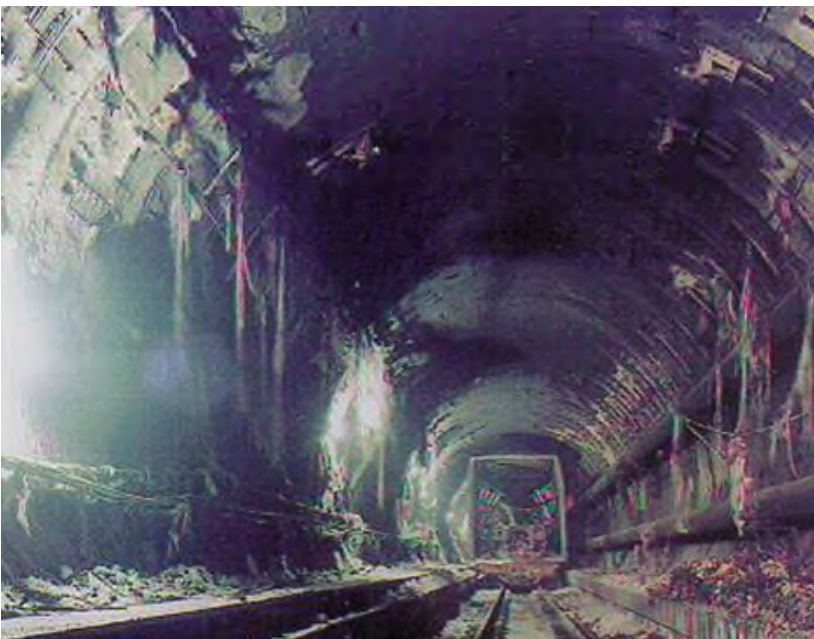
Pre-cast tunnel segments after the fire in the Channel tunnel
