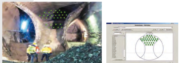
Figure 34 Tunnel face with monitoring patches (left), monitoring patches in the processing software (right).
