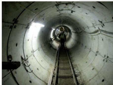
Figure 29 : Segmental lining of macrosynthetic fibre reinforced TBM tunnel
