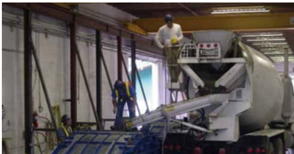
Figure 1a : Concrete delivery by concrete mixer for static mould system.
