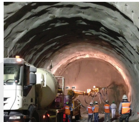
Spraying concrete at the tunnel face.
