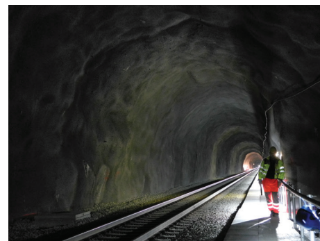
Figure 6 : Recently constructed PSCL tunnels in Norway. Right: The Holmestrand rail tunnel, constructed 2012-2015, portion in mixed face with soil and hard rock, with waterproof PSCL in the foreground and the interface to the traditional concrete segment waterproofing shield system. Left: Gevingås rail tunnel, constructed 2009-2011; meta-greywacke (meta clay/sandstone), groundwater table approximately 80 m above the tunnel crown, drained invert (Photos: Karl Gunnar Holter)
