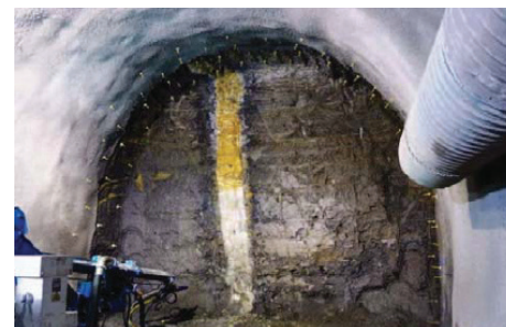
800 mm wide dyke in the tunnel face.
