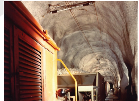
Vereina tunnel, single-track D&B section.
