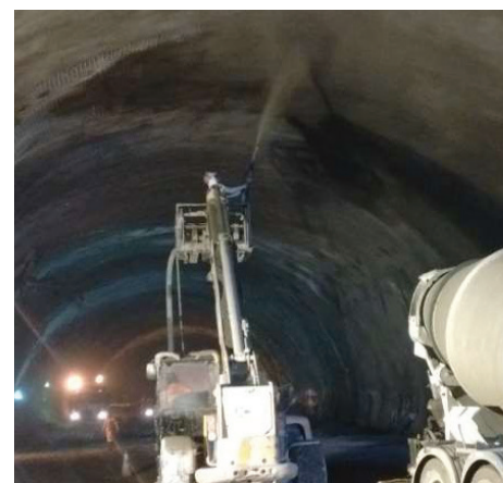
Serra do Cafezal T2, sprayed concrete lining.
