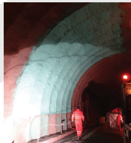
Rivarolo tunnel, application of the spray applied waterproofing layer.
