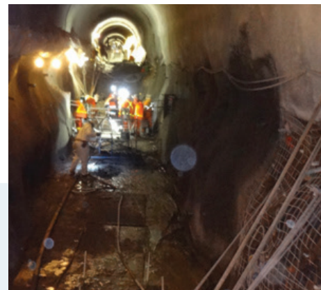
Excavation of a rock trap
