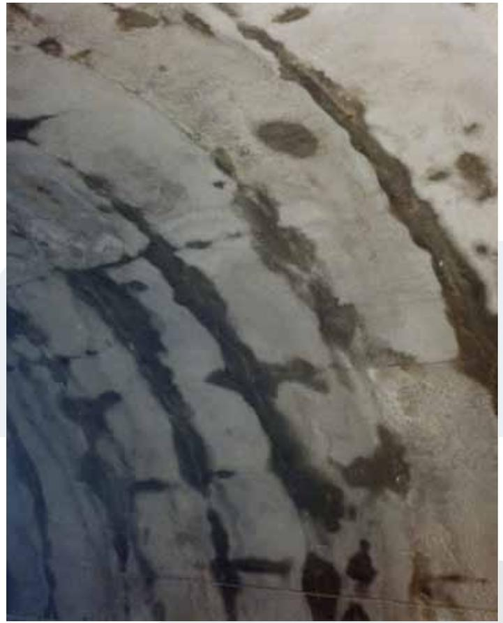
**Figure 1: Example of water ingress through a sprayed concrete lining**
