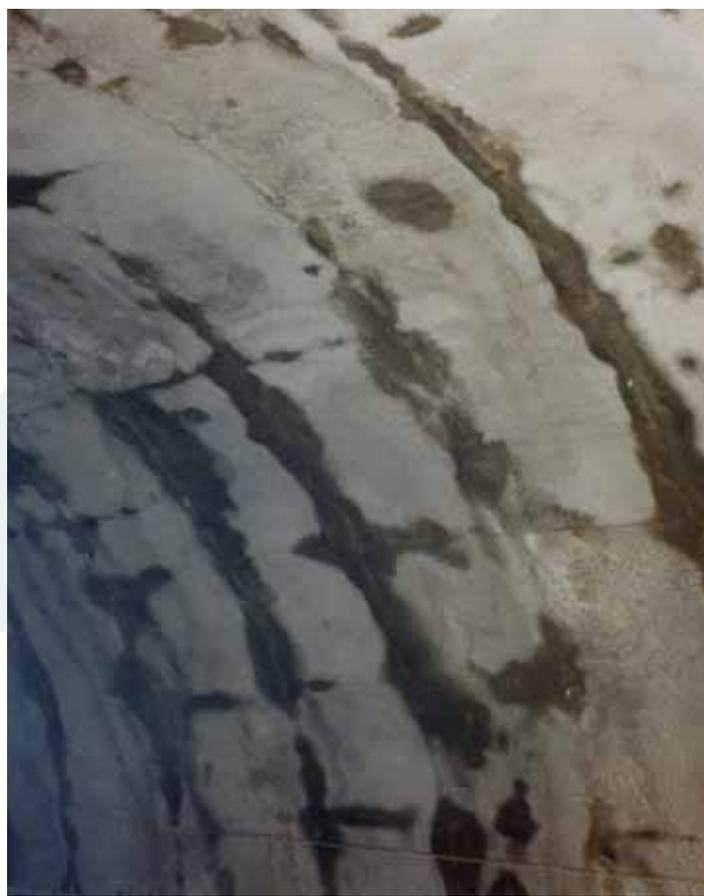
**Figure 1: Example of water ingress through a sprayed concrete lining**
