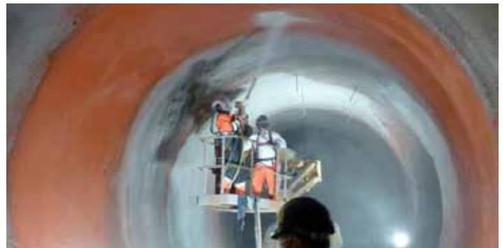
**Figure 7: Two colour application of waterproofing membrane (1st coat orange, 2nd coat white)**
