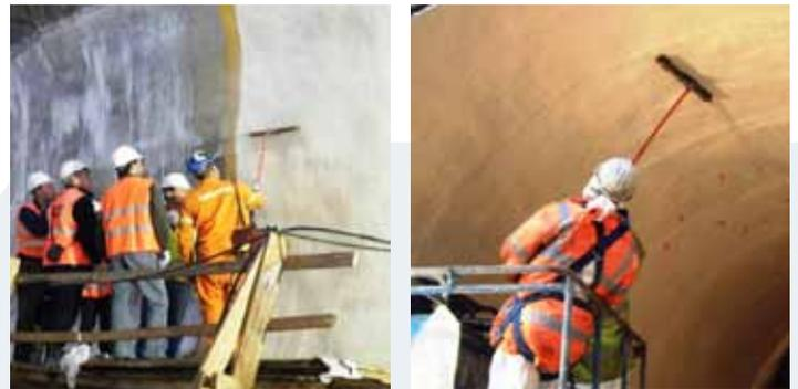
**Figure 10 : Example of integrity testing to detect and repair pinholes, voids and other defects in membranes**
