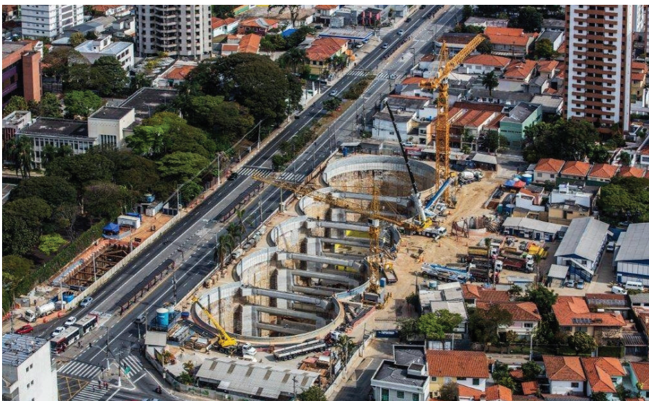
Multi-secant large diameter shafts at Brooklin Station
