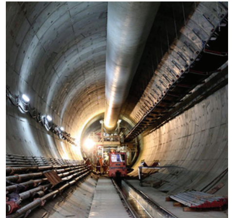
View of the segmental tunnel lining
