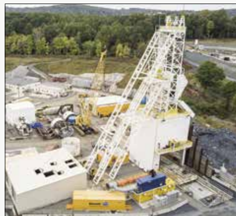
Hard rock TBM assembly on the Delaware Aqueduct bypass in the US
