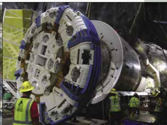
Hard rock TBM assembly on the Delaware Aqueduct bypass in the US
