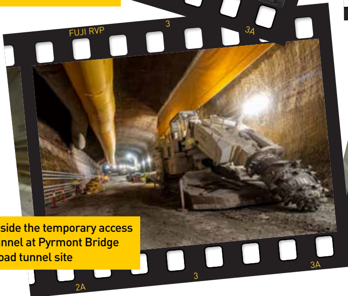
A 135 tonne roadheader excavates sandstone
