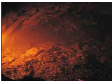
The collapse near the junction of the access tunnel and the main tunnel on Pir Panjal
