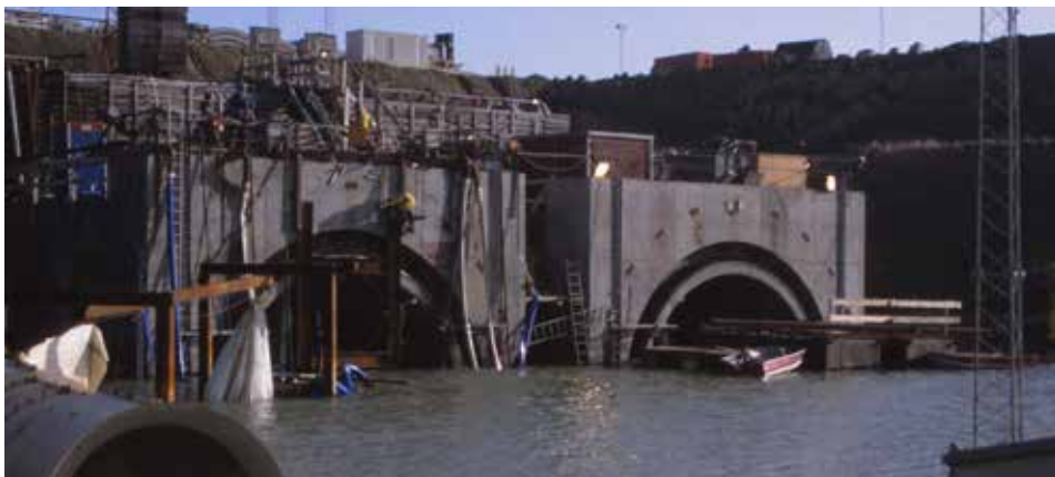
The inundation of the Storebaelt tunnels also flooded the TBM launch pit on Sprogø Island
