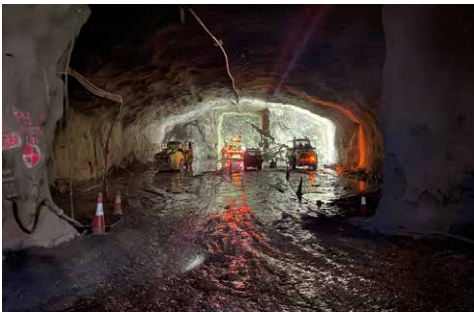
Drill and blast cavern heading
